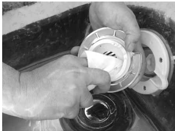
Clean back of screen Jet with same soft brush or cloth. Rinse with cold water
