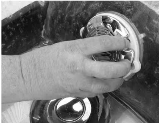
Remove screen by turning counter-clockwise.
